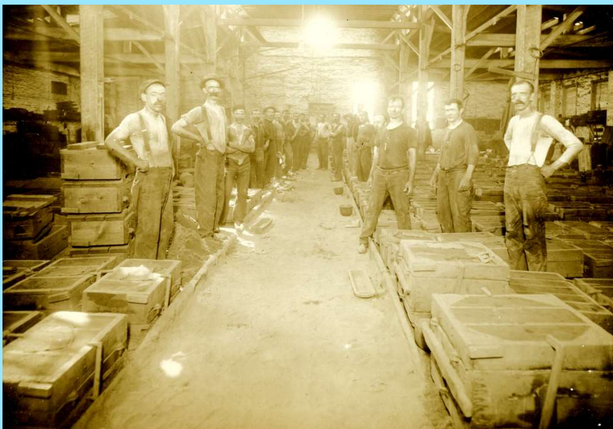
Molding room at Phillips & Clark Stove Company
