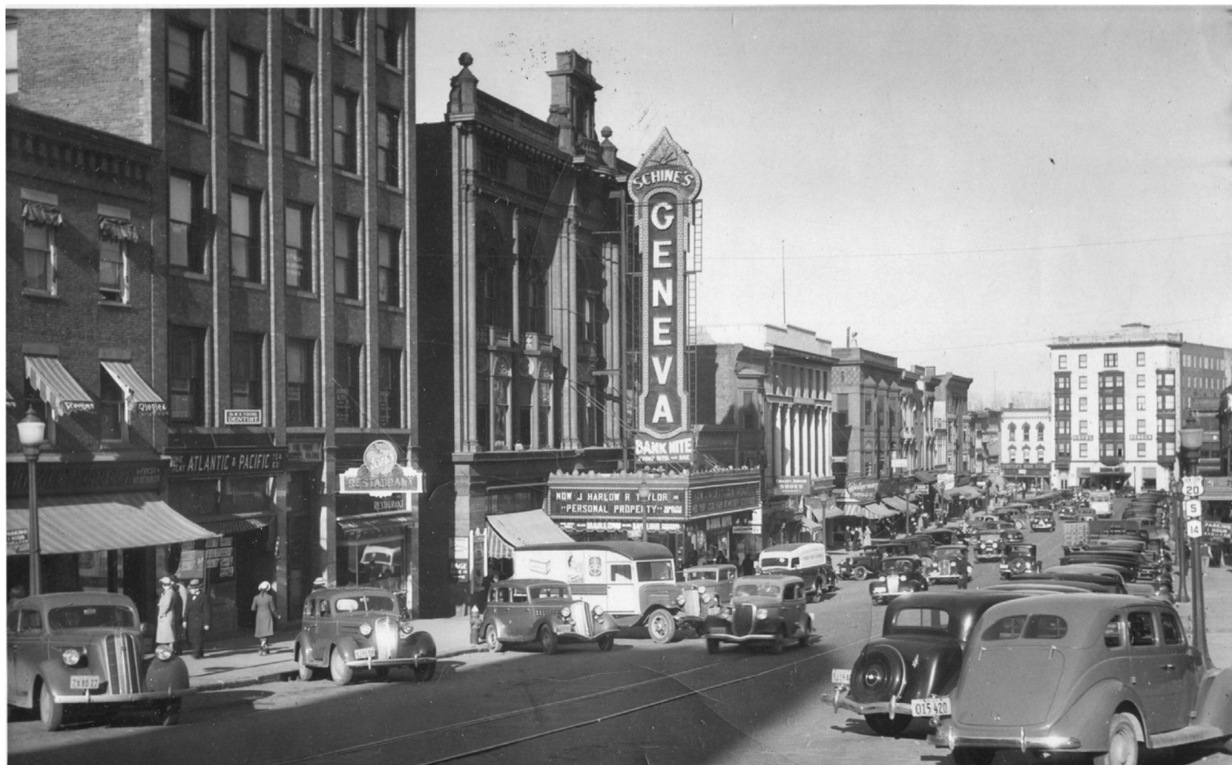
Schine's Geneva Theatre was the shining star of Geneva. Its marquee would change in style every so often as seen in this 1937 photograph looking down Seneca Street. Courtesy of Historic Geneva.
