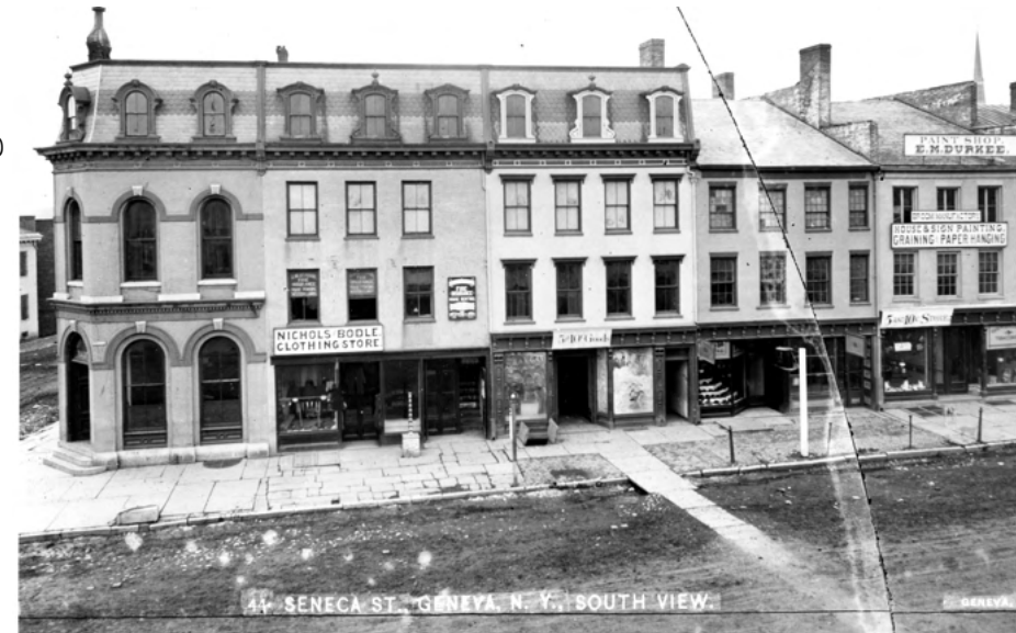
southwest corner of Seneca and Exchange
