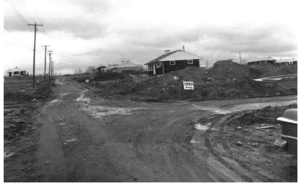
The Arbors construction of West High Street
